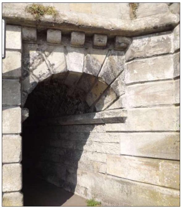
Figure 21 Detail of the pedestrian arch of Trent Lane Bridge. Stone is used for the more consciously styled buildings and structures
