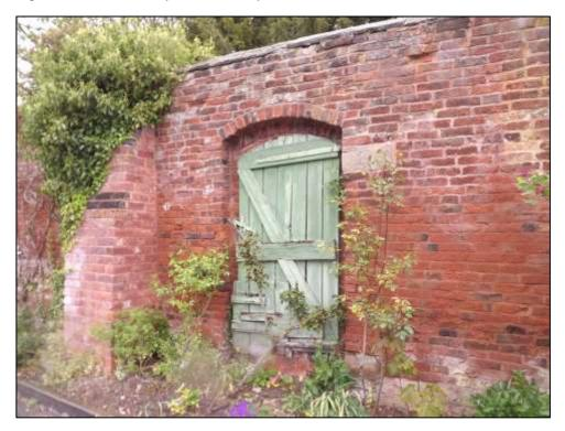
Figure 37 The continuation of Abbey House boundary wall at Abbey Gardens. The remaining plank door with original iron strap hinges is in need of repair but adds charm to the walling
