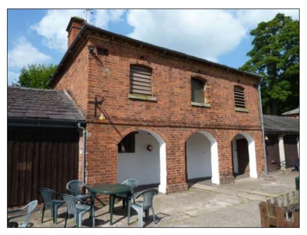
Figure 79 Central block with brick piers. Stone piers to the right indicate the bays were open at the front.
