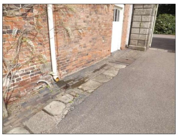
Figure 59 Stable block (south courtyard) Historic paving is visible under the later surface
