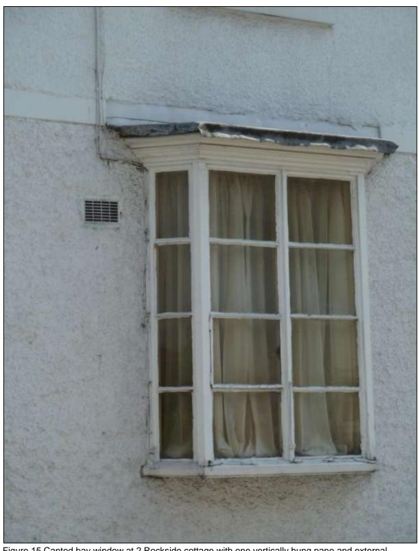
Figure 15 Canted bay window at 2 Rockside cottage with one vertically hung pane and external fastening.
