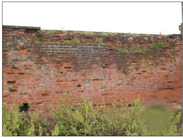
Figure 70 Vegetation and spalling on the brick faces
