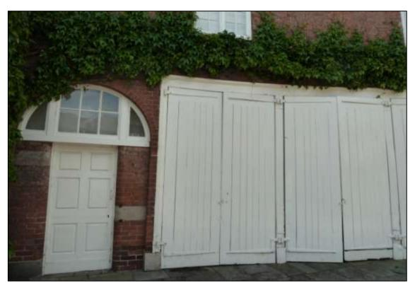
Figure 58 Service courtyard, west facade. The retention of plank doors with L- shaped wrought iron hinges and varied fenestration reflects the former functional use of this courtyard.
