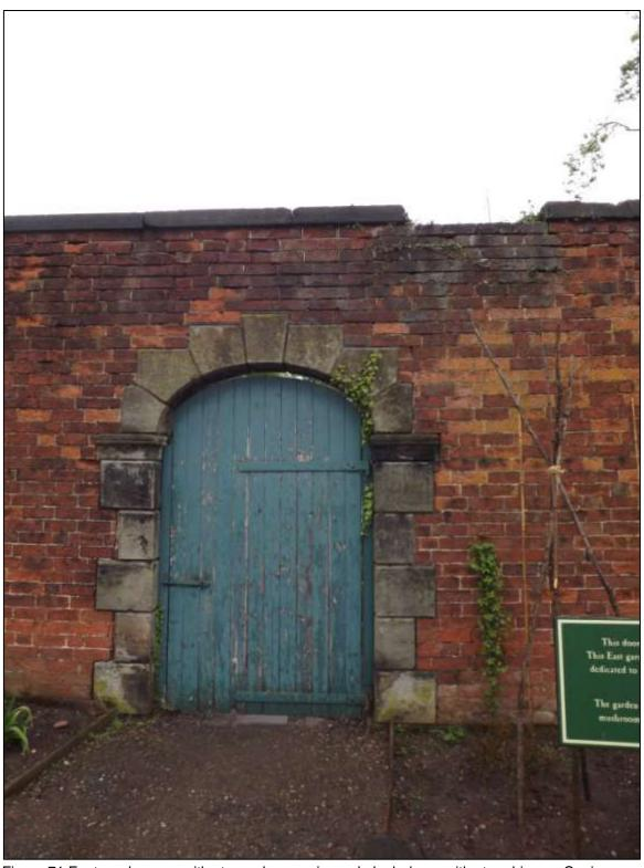
Figure 71 Eastern doorway with stepped voussoirs and plank doors with strap hinges. Copings are missing.
